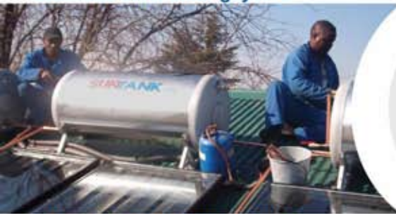
In-house installation technicians
